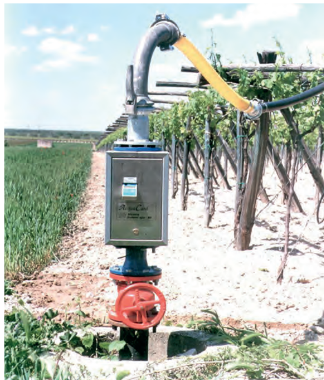
Irrigation hydrants for automatic, selective and controlled water distribution, equipped with a hydraulic device coupled with electronic components. The quantity of water supplied can be programmed by an electronic card assigned to farmers
